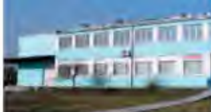
Production centre for machines and equipment in Slovakia
