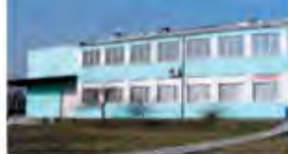
Production centre for machines and equipment in Slovakia
